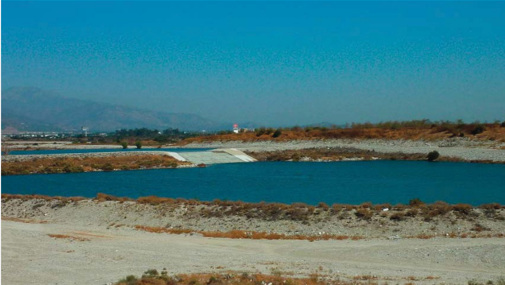
The Santa Fe Spreading Grounds are operated and maintained by the Los Angeles County Flood Control District.
