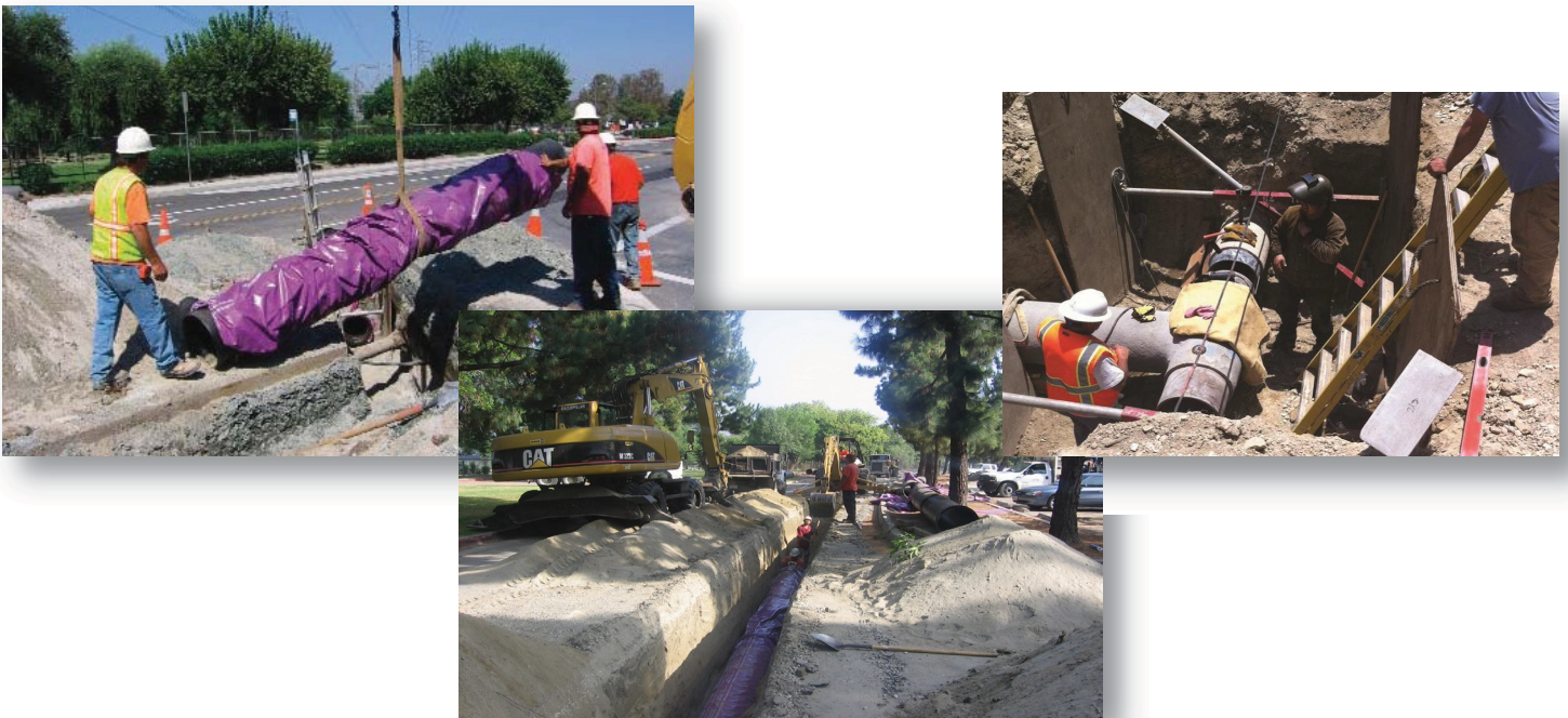
Installation of Recycled Water Pipeline
