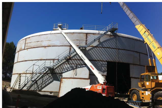
Construction of 2 Million Gallon Storage Tank for photo in upper right.
